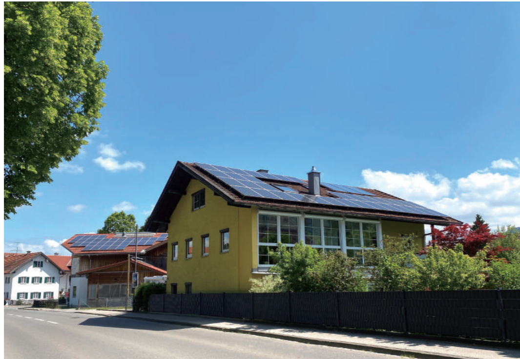
12 Residential ESS Project in Europe
